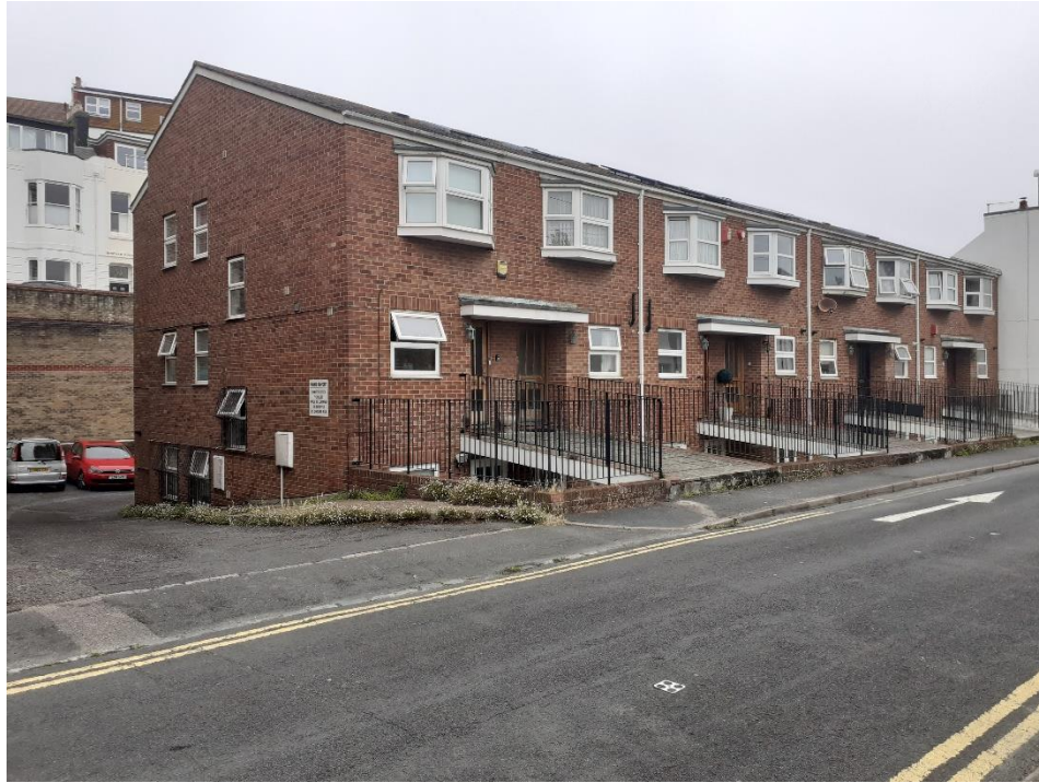
Looking west over Centurion Road, brick-built properties are 55-69 Centurion Road. Driveway to south is access to rear car parking area,
