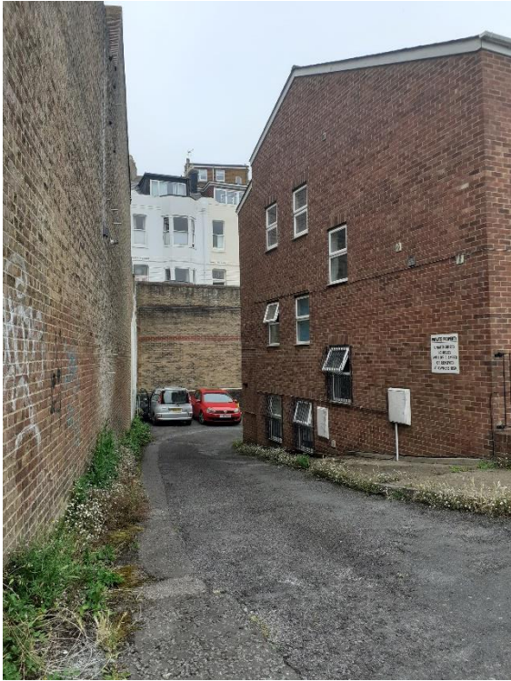
Access from Centurion Road to rear car parking area and garages.
