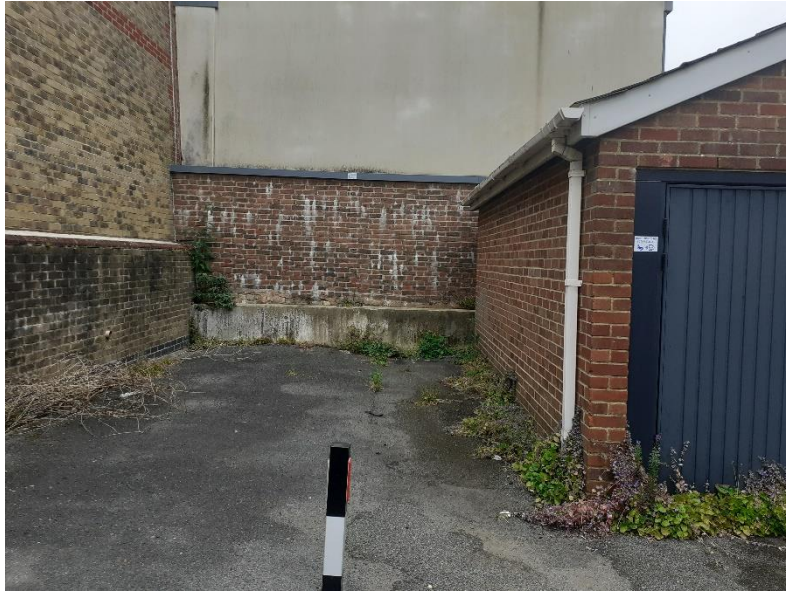
Space to the west of the existing garage
